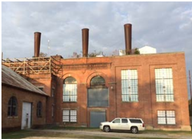
The old Kinston power plant, new home of Social Beverage Company.
