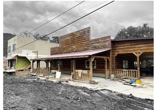
Town of Hot Springs—Repair of Bridge Street sidewalk and stormwater improvements
