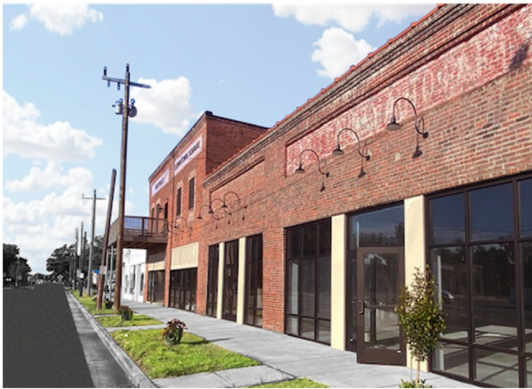
Town of Maysville—Restoration of old buildings downtown Main Street
