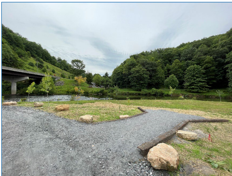
Photo 3: Newly developed river access on the South Fork of the New River near NC-163
